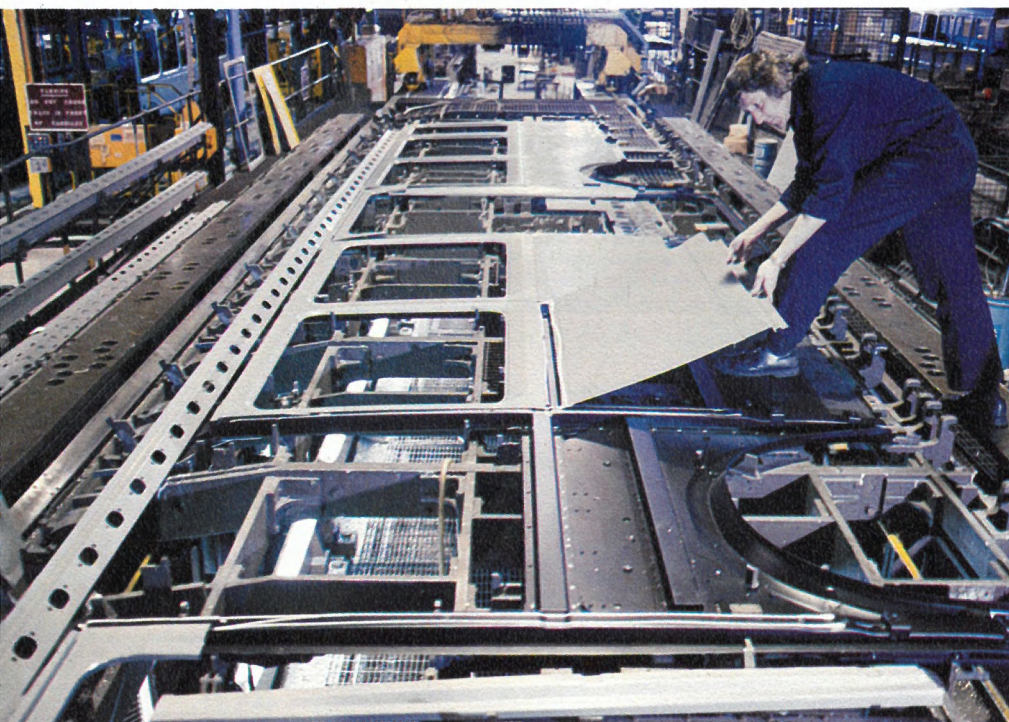
Jig built construction of National side frame
